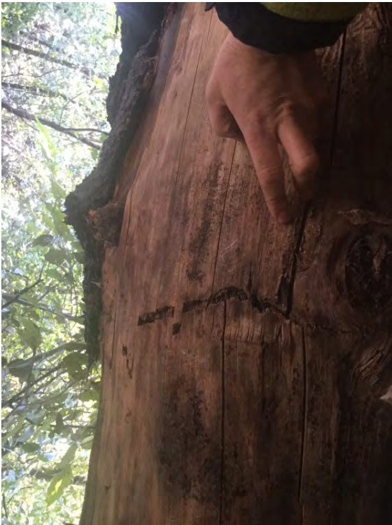
Stringer 12 - cracked midspan
